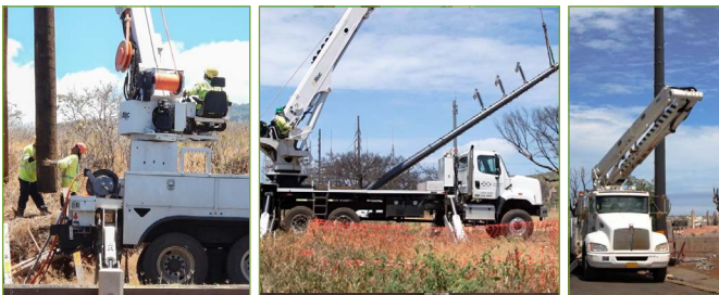
Crews are working to replace, upgrade, and test poles.
