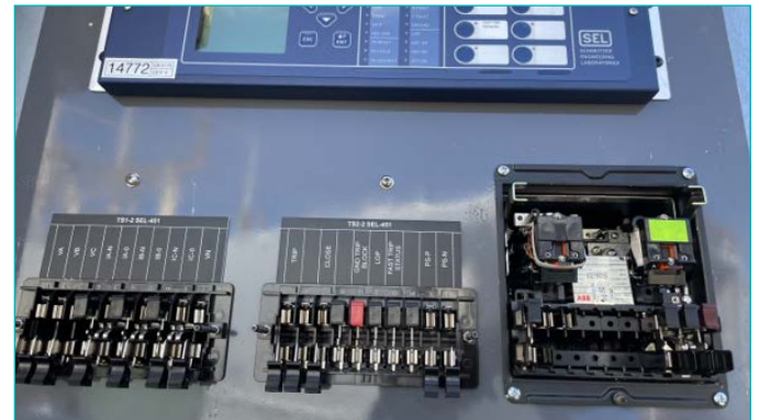
Enhanced Fast Trip and Reclose Blocking equipment helps detect disturbances to Hawaiian Electric equipment and alert the team of the need for a visual inspection.
