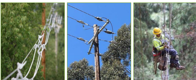
Crews work to install covered conductors on Hawaiian Electric equipment.
